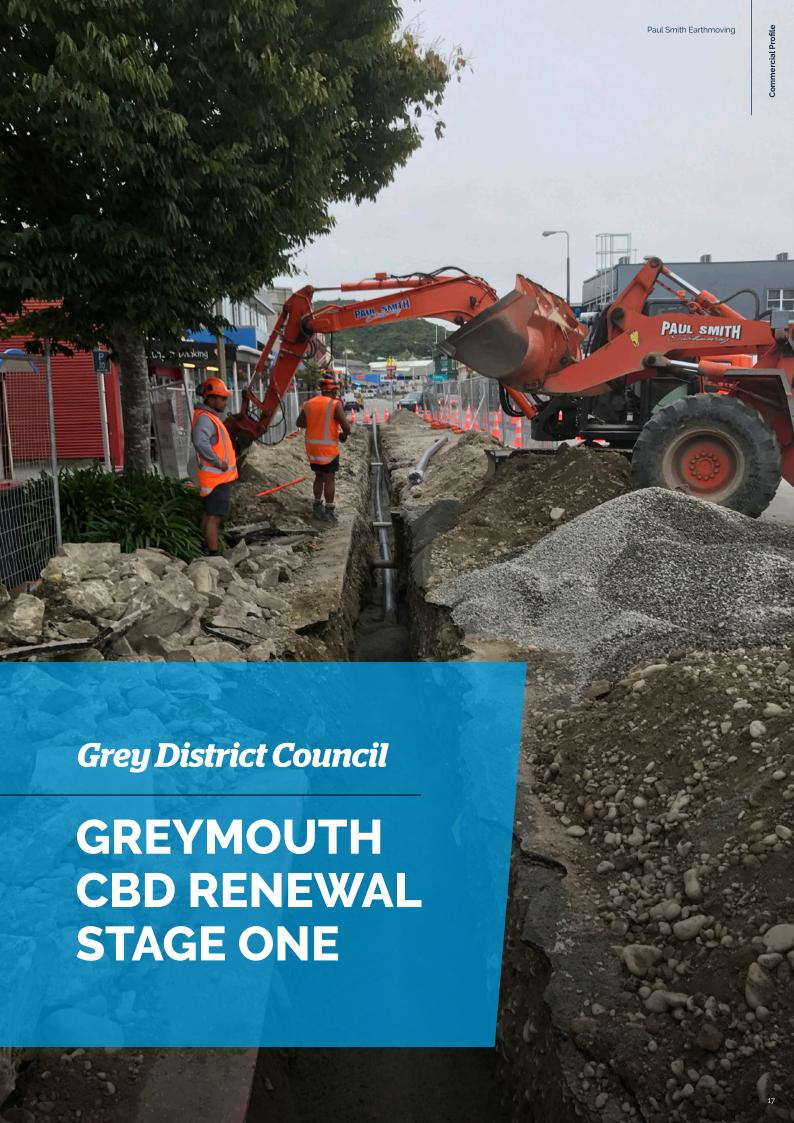
CBD renewal project consisting of excavation, removal and replacement of the existing road pavement, kerb and channel and footpaths and installation of interlocking pavers along with all associated ground and pavement preparation works. Water and stormwater renewal and installation works.
