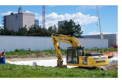
Civil works project consisting of bulk excavation and fill earthworks for new building platform, earthworks and landscape bund construction, stabilised construction access, full construction of new roading, full construction of new pavements, kerb and channel installation and all associated drainage.
